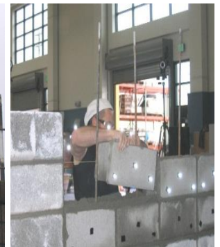
Photo 2 - Laying H-Block around rebar
