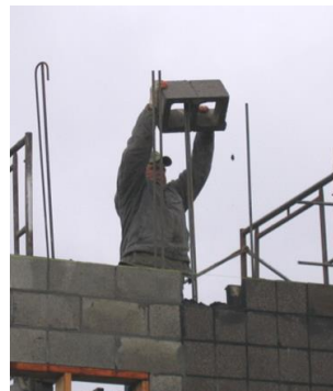
Photo 1 - Laying CMU over rebar
